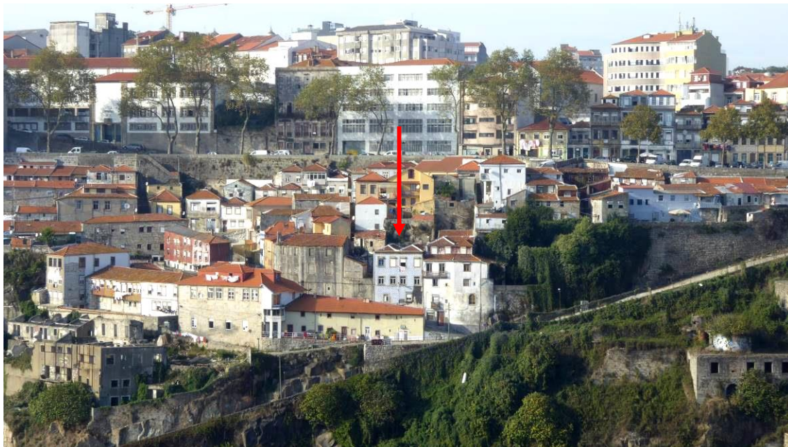
Figure 4 – Building photography taken from the opposite bank of “Rio Douro”.
